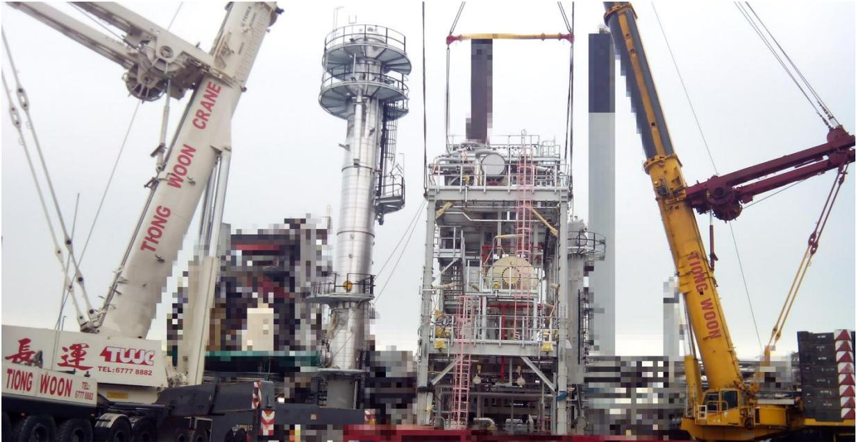
Our Demag AC500-2 (500 Tons) and AC700 (700 Tons) Mobile Cranes were deployed and configured in HASSL (Main Boom Side Superlift) for the tandem lifting of Modules for the heavy lifting operation.
